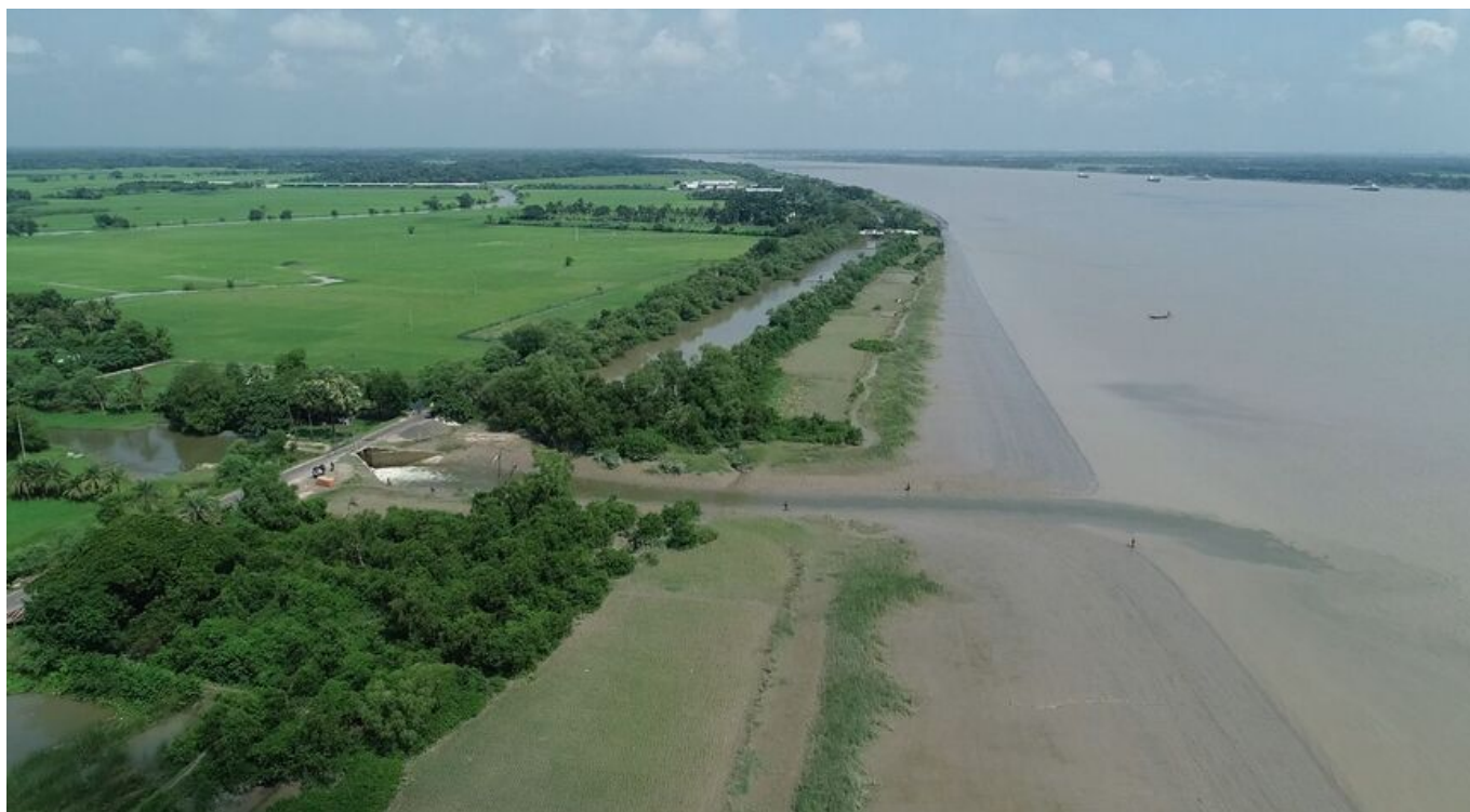
Photo C.1 A regulator draining excess water from Polder 31-part into the Kazibacha River
