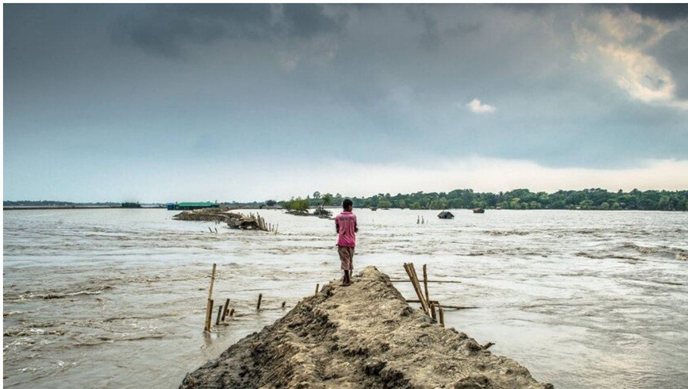
Photo 11.1 The third breach in the realigned embankment (August 2015)
