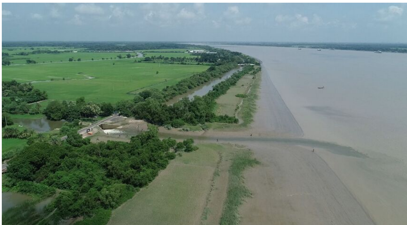
Photo 3.1 A regulator draining excess water from Polder 31-part into the Kazibacha River
